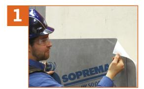
Peel off the top portion of the silicone release film and adhere the membrane to the substrate, making sure the membrane is well aligned.
